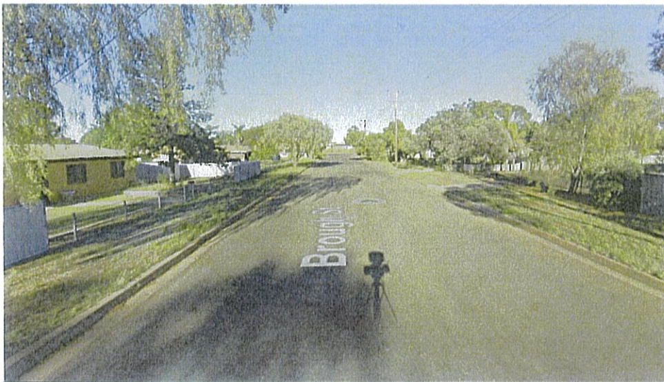
Photo 2: 57 Brough St, Cobar: Access and Road. Source: Google Maps
