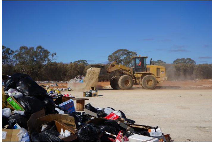
Step 2- Spread capping soil across face of the waste
