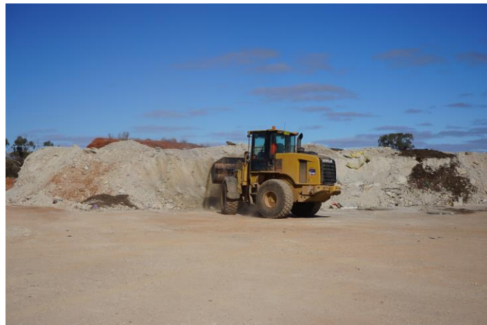
Step 1- Obtain capping soil from stockpile adjacent to waste cell
