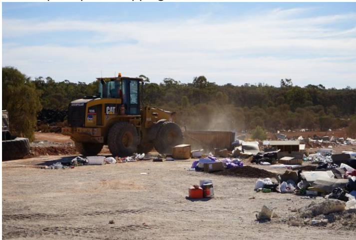
Step 3- Using rake, push soil into waste and continue this process until waste covered with soil
