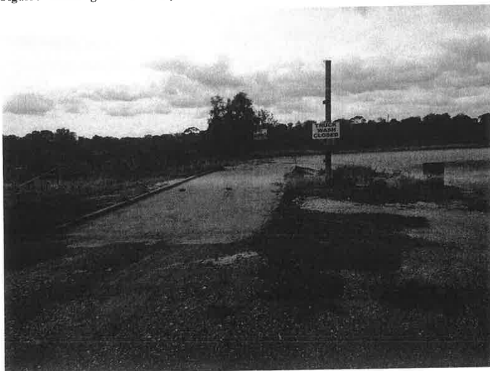
Figure 2 – Existing truck wash bay
