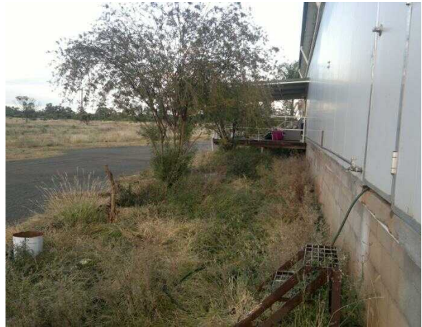
Figure 4.2. Northern side of the existing building
