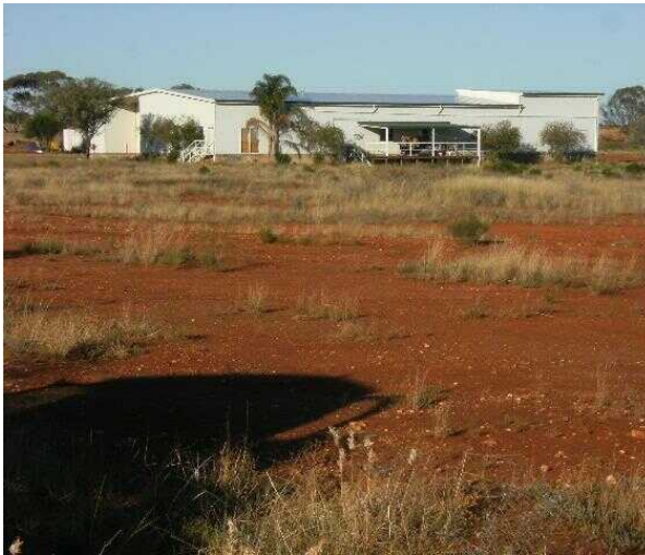
Figure 4.1. Looking south toward the existing building
