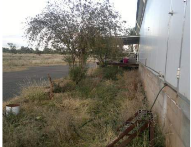
Figure 4.2. Northern side of the existing building
