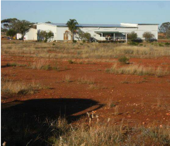
Figure 4.1. Looking south toward the existing building
